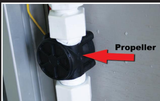
*A propeller measures the volume of water passing through*
